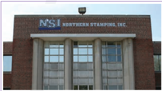
Northern Stamping Inc exterior signage install
