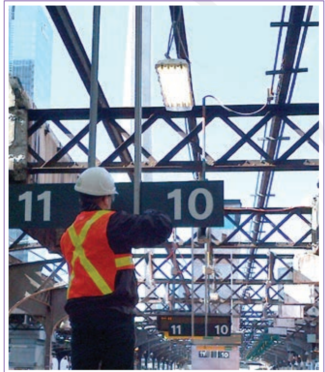
MetroLinx platform signage install
